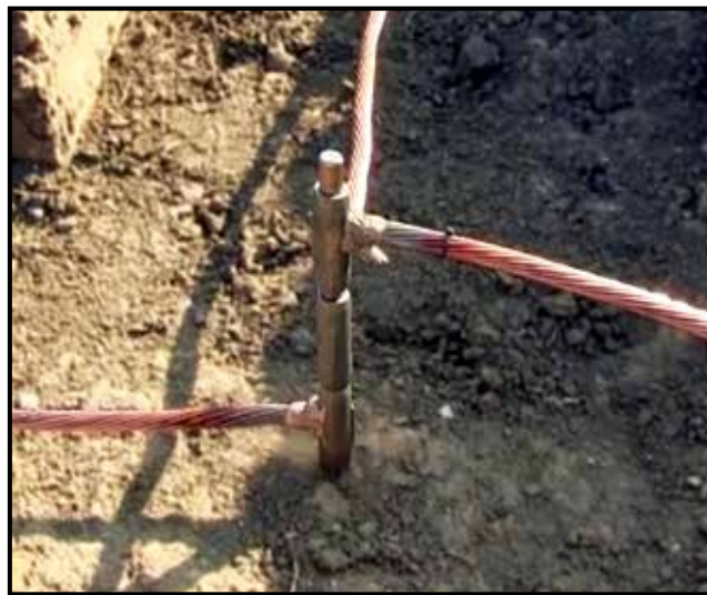
QuikTap stacked for multiple direction application.
